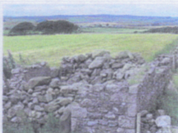
Ruined Episcopal chapel from 18th century where the clergymen conducted their services leading to imprisonment
